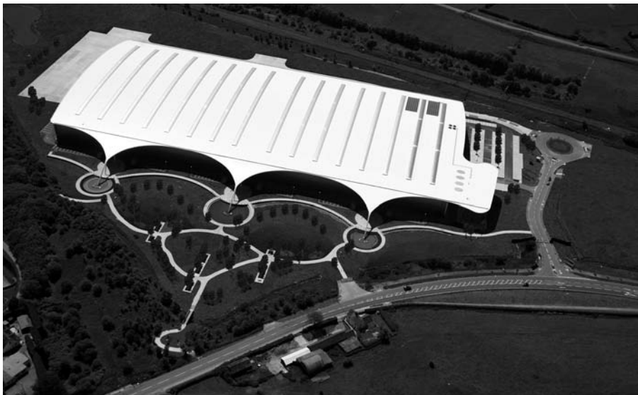
Figure 8.4 Chatterley Park Distribution Centre
